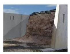
Timber contacting silage should not be treated with preservatives and silage acids will corrode concrete or steel over time. Round bales lined with plastic have also been used for bunker storage walls, but this is typically a temporary solution.
