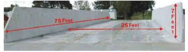
than the width of tractor. From front and back sides bunker should be open. Out of front and back side, concrete floor is constructed up to 15 feet.
